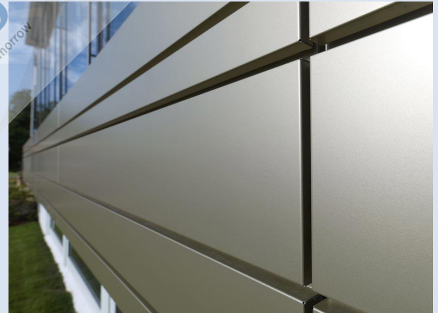
Example of outer building application
